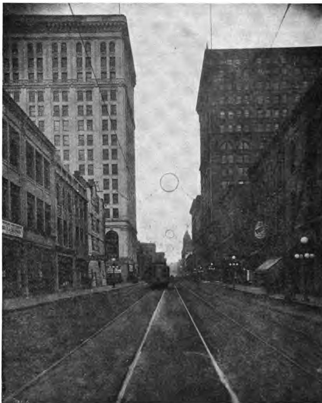
Robert Street, St. Paul, after widening. This improvement was made without cost to the city except for street reconstruction
